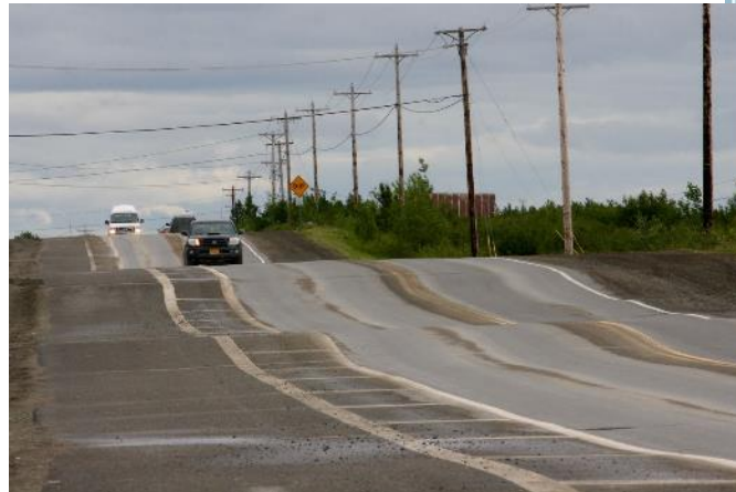
Roads affected by melting permafrost.
